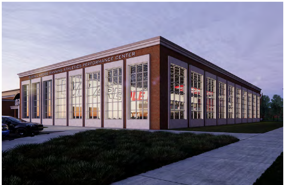
Renovation began on the $45 million Olivia and Archie Manning Athletics Performance Center in January 2022 and was completed in July 2023.
