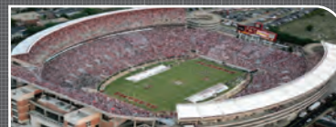
CAPACITY: 92,138 NORTH END ZONE UPPER DECK AND CLUB LEVEL ADDED
